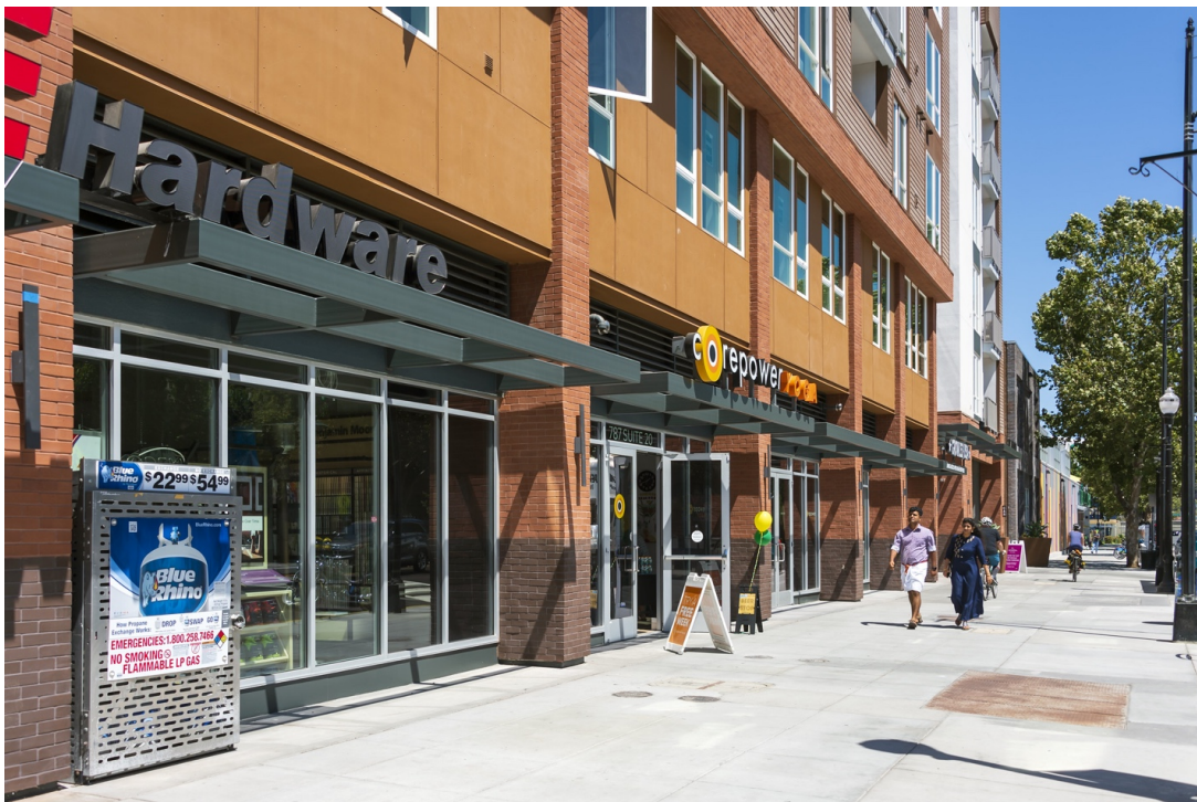
Modera the Alameda is one project that has pioneered a small amount of commercial space on the second floor.
